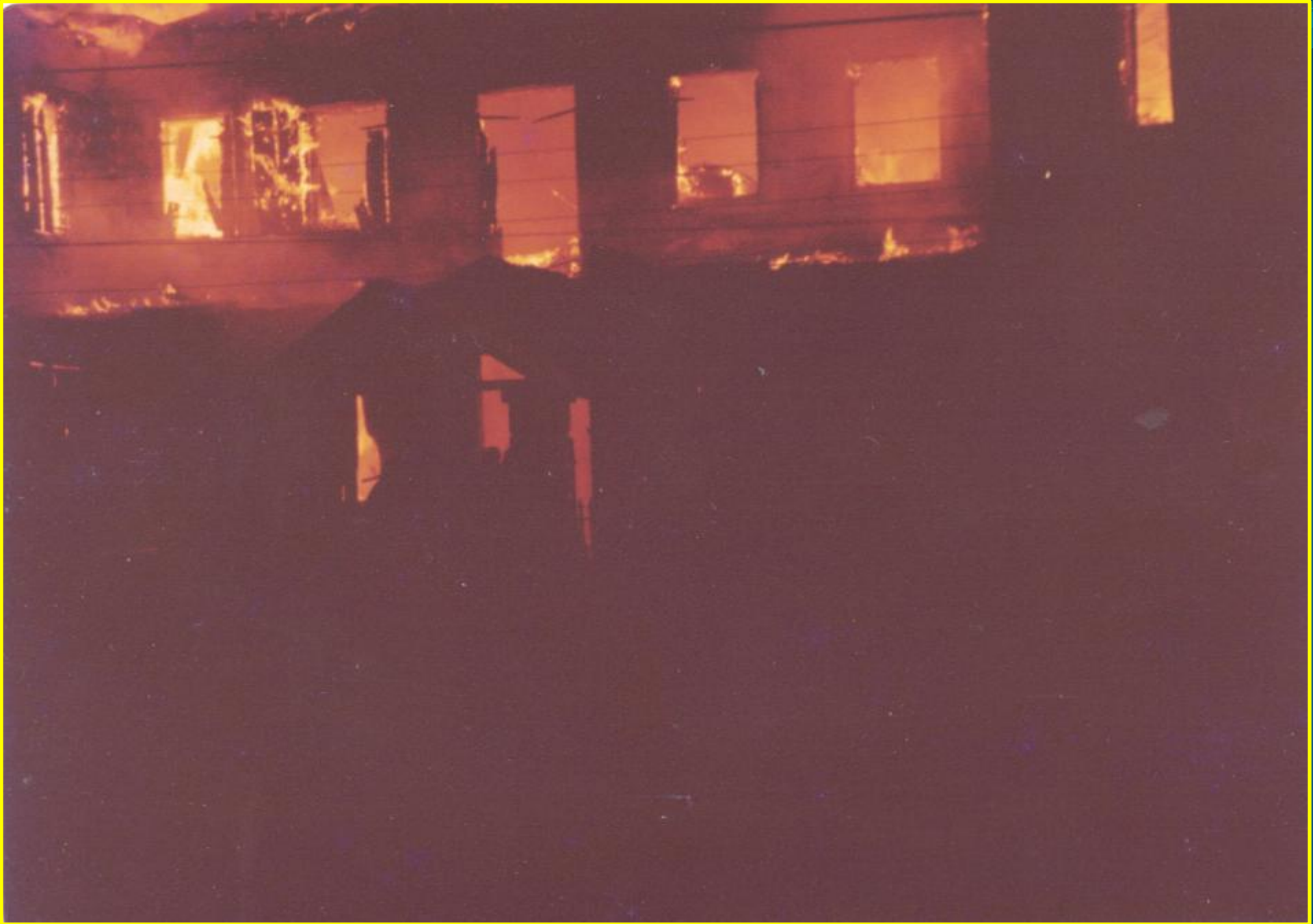
The Registry and High Court Building ablaze, 16 th June 1979. Arson???
